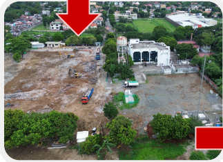
Start of Construction November 2023
