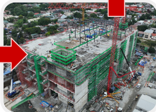
Structural Top-off November 2024
